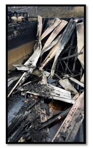
garden hoses. This water use created a high water demand on the water system all at once, causing a siphoning effect in both the good and burned tank. Charred wood and other debris in Reservoir #1 was quickly drawn in to the pipes throughout the water system in town.
